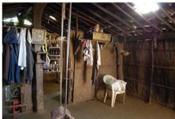
Photo 8: Timber pillars and beams, bamboo purlins, hay and hemp used as walls.
