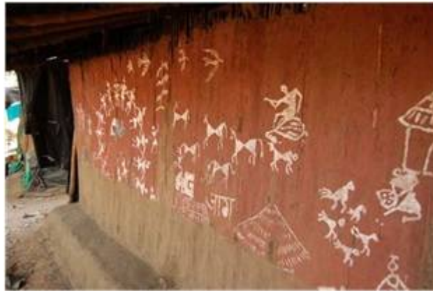
Photo 5: Bamboo purlins and mud plaster.
