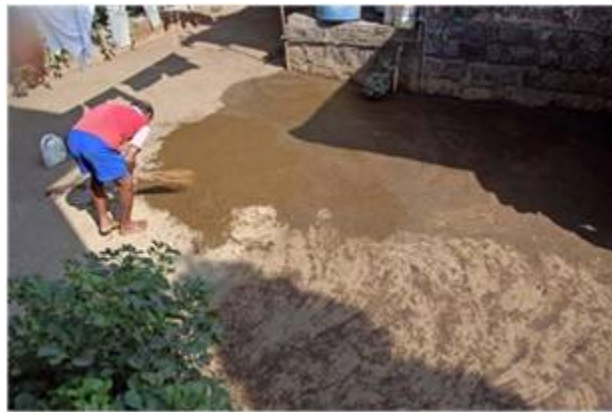
Photo 7: Stone walls and mud floor.
