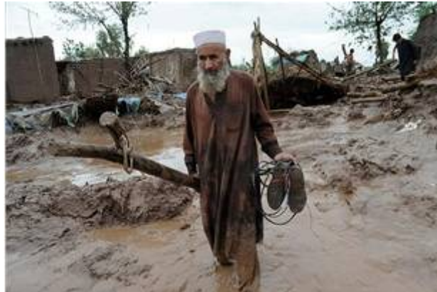
Photo 1: Mud plaster adversely affected by rain.
